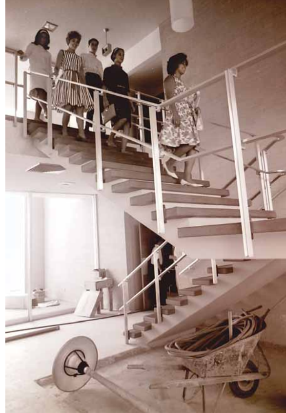
Students in Scott Hall, still under construction, August 15, 1964.
