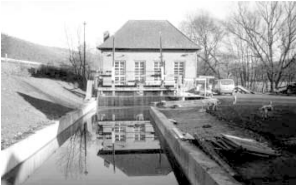
The Voelkelt's hydroelectric power plant. The plant was reactivated on November 30, 1999, after standing still for almost five years.
