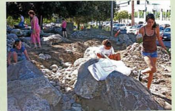
Pitzer students building a dry streambed in the new garden they designed in front of two popular lecture halls. Photograph by Joe Clements
